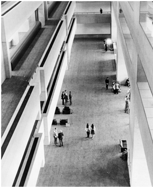
Fig. 6 – View of the central interior gallery with the post-tensioned bearing walls that support the North Facade (on right)
