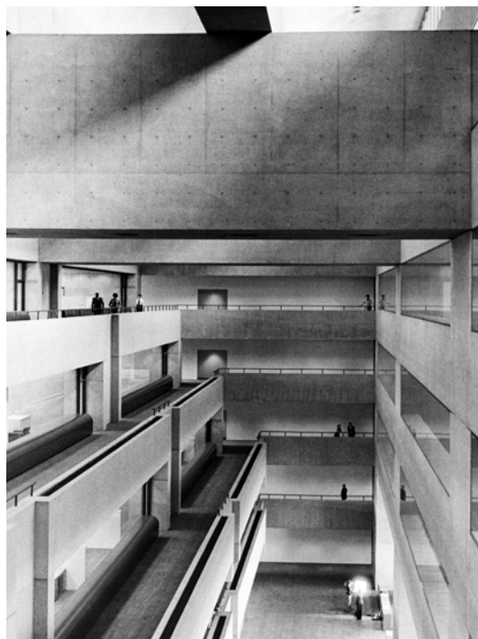
Fig. 7 – View of the cantilevered box beam
