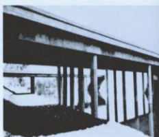
Fairborn, OH • Highway Bridge Deck
