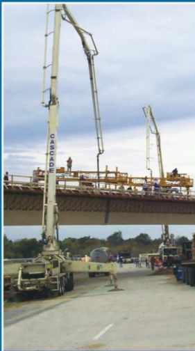
Michigan DOT Bridge Construction Grand Rapids, MI
