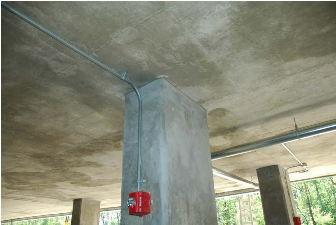
Figure 5 – First Level Slab-Column Joint Looking West
