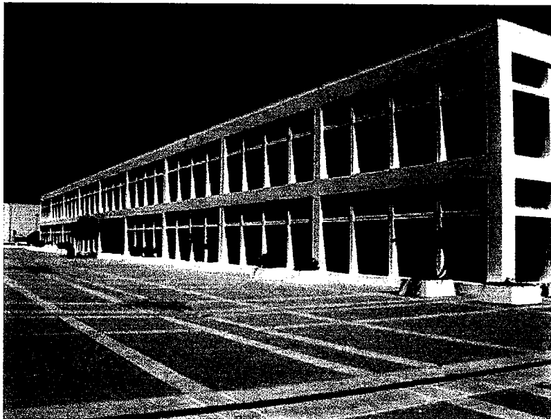
South Elevation Building R6 – Looking Down 439 ft. Length at Plaza Level
