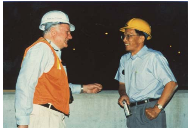
Fig. 4 - Teng Li (right) on the jobsite during a night-time pour in 1998 with Edward Rice, one of the original developers of shrinkage compensating concrete and 2005 recipient of the PTI "Legends of Post-Tensioning" award.
