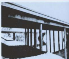
Fairborn, OH • Highway Bridge Deck
