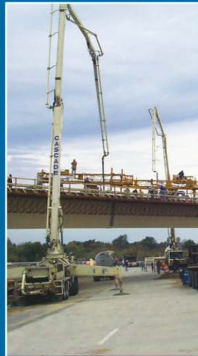
Michigan DOT Bridge Construction Grand Rapids, MI
