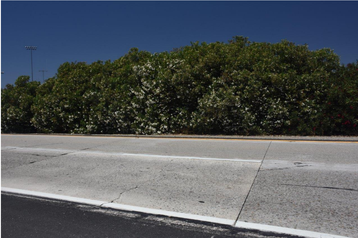
Figure 8. Highway SR-126 near Ventura, CA showing an original 18-19 ft thin slab (conventional concrete) placed in 1972 that developed a transverse fatigue top down crack (this result is common as these thin slabs cannot carry this many heavy truck axle loads).
