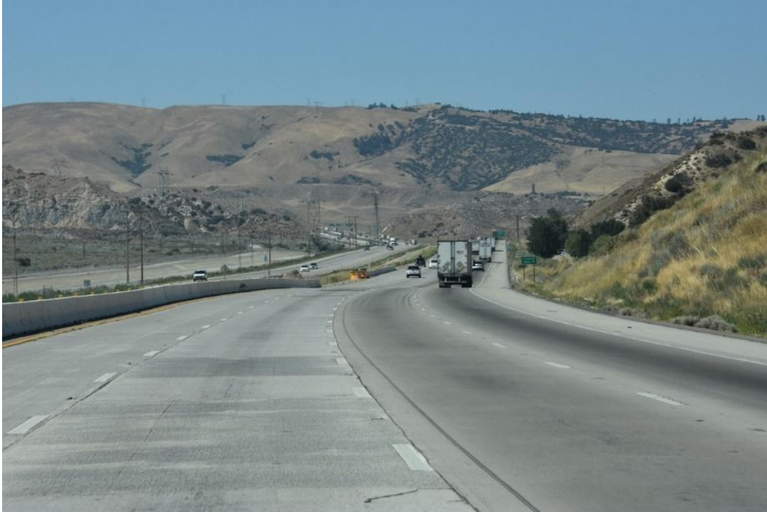
Figure 9. Highway I-5 NB direction (PM 76-88), northwest of Los Angeles showing original inner #1 lane (left) and inner #2 lane with several “Individual RSC” slabs placed in 2005.
