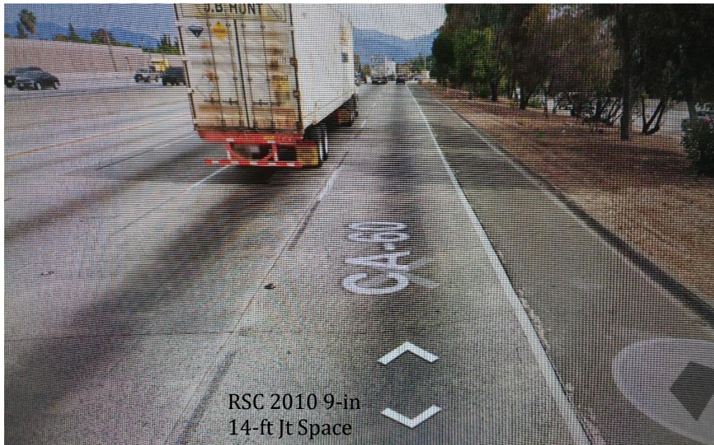
Figure 20. Photo (from Google Maps) of a “Lane Replacement RSC” section on CA-60 located in Los Angeles Co., CA constructed in 2010.
