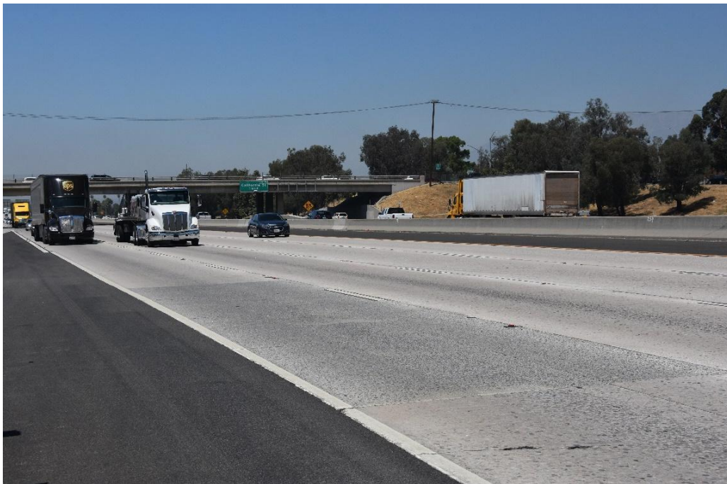
Figure 12. Highway I-10 EB direction (PM 0-39), near San Bernardino showing two 14-year old “Individual RSC” slabs in Lane #4 (outer lane).
