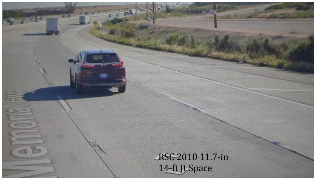
Figure 21. Photo (from Google Maps) of a “Lane Replacement RSC” outer lane section of I-15 located in San Bernardino Co, CA constructed in 2004.
