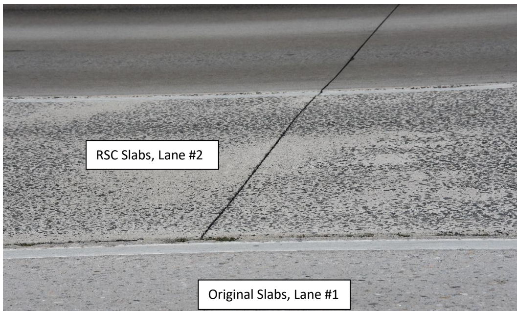
Figure 10. Highway I-5 NB direction (PM 76-88), northwest of Los Angeles showing a transverse joint between two 13-year old RSC slabs (Note that variation in mix color did not create any cracking or disintegration).
