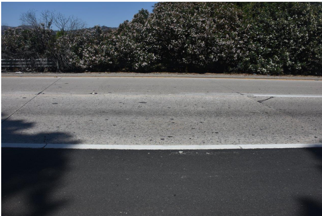
Figure 17. Highway SR 126 (PM 0-13) near Ventura showing a RSC slab placed in outer truck lane in 2006 that has developed a top down transverse fatigue crack.
