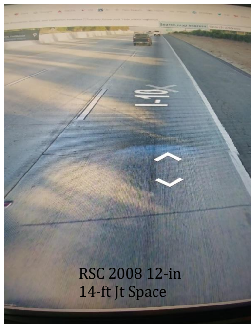
Figure 23. Photo (from Google Maps) of a “Lane Replacement RSC” outer lane section of I-10 located in Riverside Co, CA constructed in 2008.
