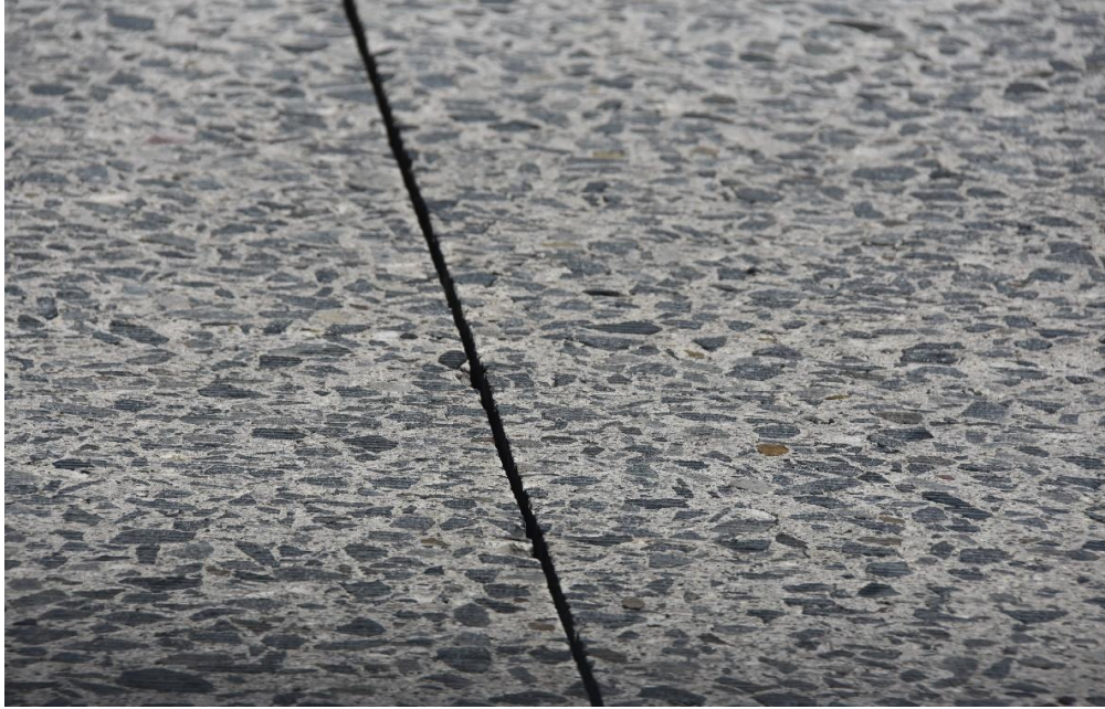
Figure 13. Highway I-10 EB direction (PM 76-88), near San Bernardino showing a closeup of a 14-year old diamond ground transverse joint “Individual RSC” slab in Lane #4 (outer lane). Very good RSC durability shown here existed at all sites.
