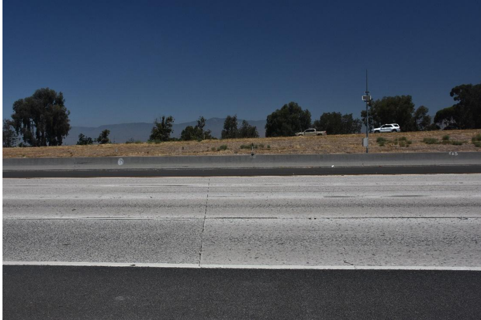
Figure 15. Highway I-10 EB direction (PM 76-88), near San Bernardino showing on the left side a 14-year “Individual RSC” slab surface Lane #4 (outer lane) and on the right an original (1970s) JPCP slab with a transverse fatigue cracking.
