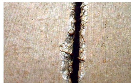
Fig. 10 – The fibrous slab also suffered spalling at its sawcut joints..
