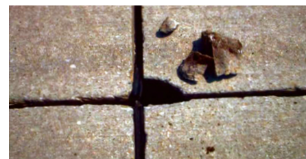
Fig. 9 – Joints in the non-post-tensioned pavement show the spalling typical of 10 years of heavy aircraft traffic and snowplow damage.
