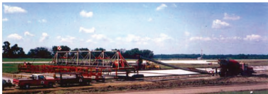
Fig. 4 – The bridge deck paver, an 80-foot truss with conveyor belts, and a truck feeding it concrete.
