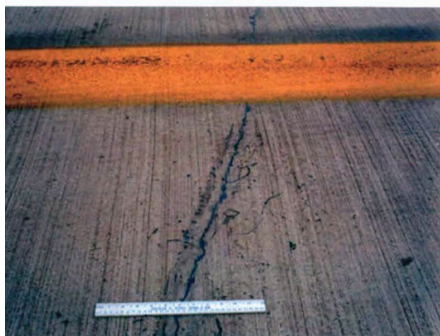
Fig. 3 – The transverse crack in the unjoined slab, repaired with epoxy, has remained closed ever since post-tensioning.
