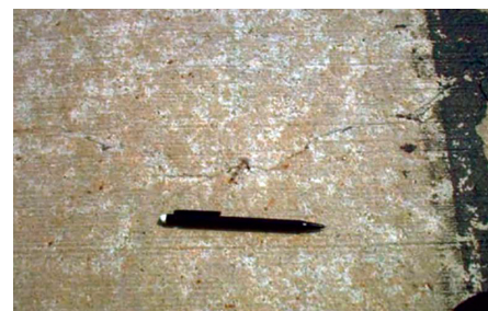
Fig. 11 – The post-tensioned pavement has cracks, but they are tight and less vulnerable to impacts that cause spalls.
