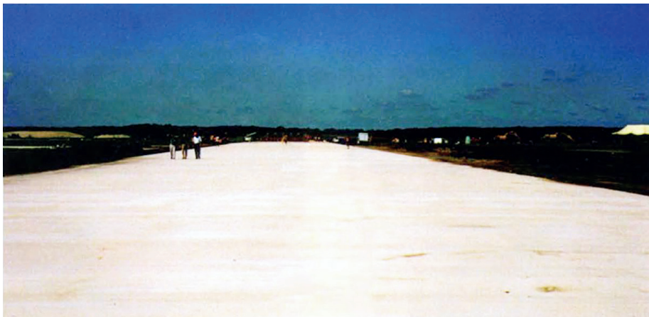
Fig. 1 – The finished 1200 foot slab shortly after pouring, probably the longest jointless concrete pavement in North America.
