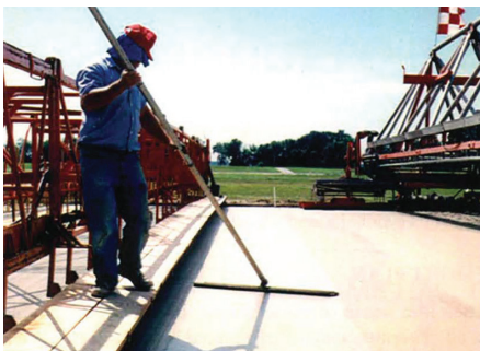
Fig. 6 – Bull-Floating Concrete.
