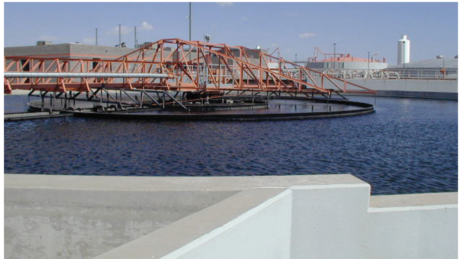
Fig. 3 – Waste Water Treatment Plant.
