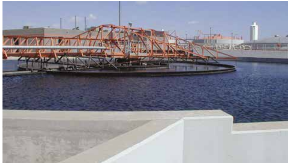
Fig. 3 – Waste Water Treatment Plant.
