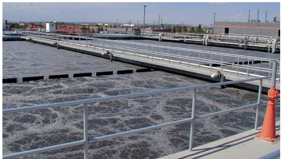
Fig. 4 – Waste Water Treatment Plant.
