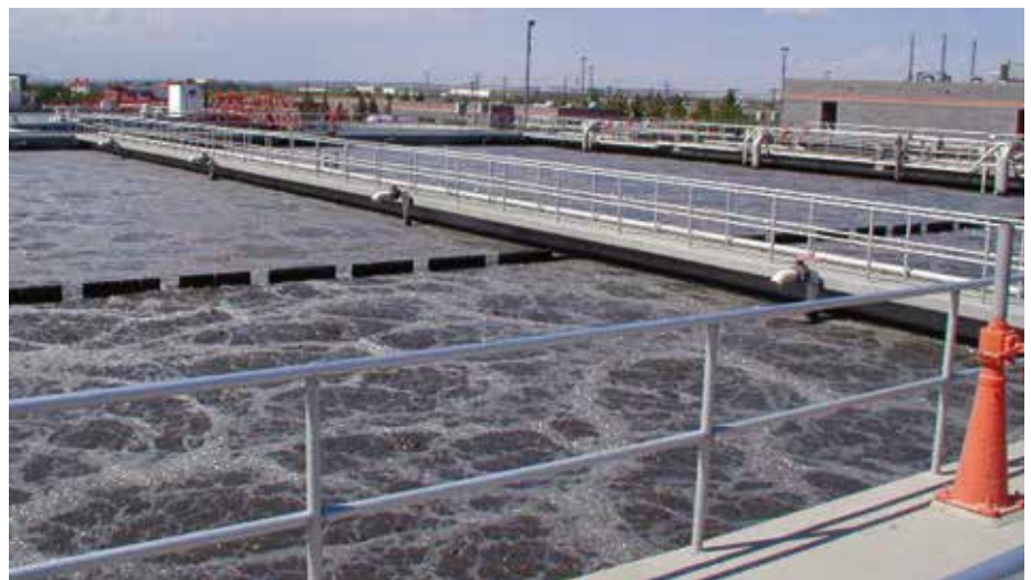
Fig. 4 – Waste Water Treatment Plant.
