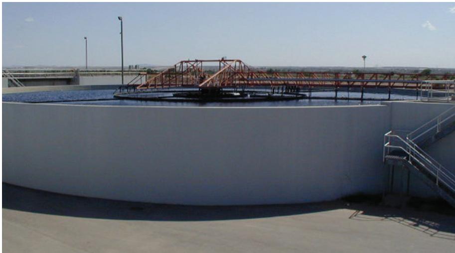
Fig. 1 – Roberto R. Bustamante Waste Water Treatment Plant.
