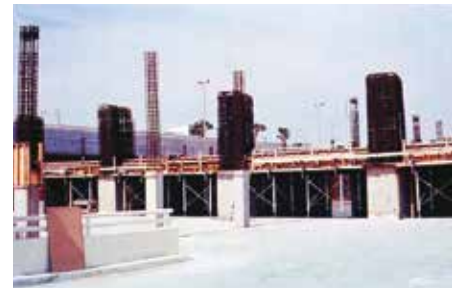
Fig. 11 – Formwork and reinforcement in place in the summer of 1998.
