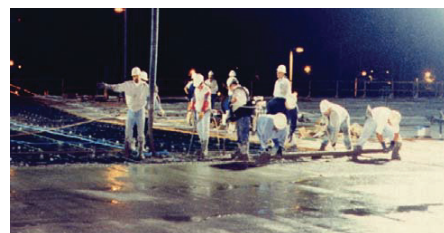
Fig. 12 – Type K concrete was placed at night to accommodate airport traffic regulations and to protect the fresh concrete from excessive summer heat.
