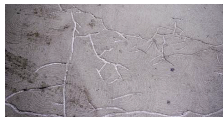
Fig. 9 – 70,000 ft of cracking in Level 1 of the original structure was routed out and sealed to eliminate water infiltrating the slabs or leaking through onto cars on Level 0 below.
