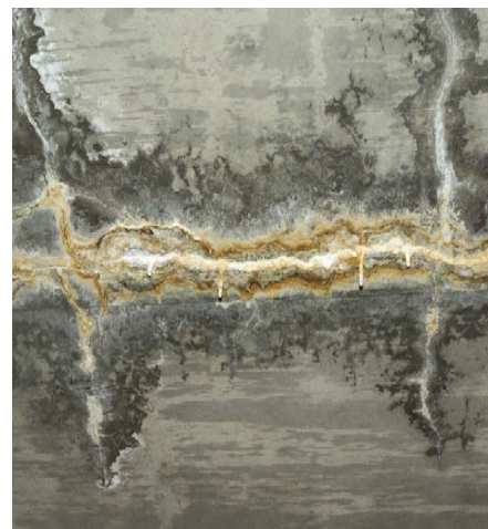
Fig. 6 – Cracks in the Level 1 deck of the original structure as seen from the underside. Water leaking through the cracks carried lime from the interior of the conventional concrete, depositing disfiguring efflorescence and dripping onto cars on Level 0.
