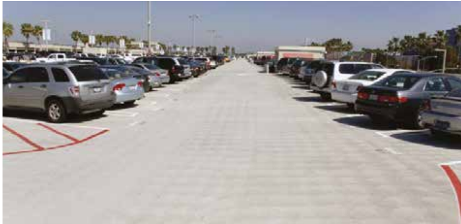
Fig. 1 – The top deck of new parking structure, made with shrinkage compensating concrete, still looks almost new after nine years of heavy use.
