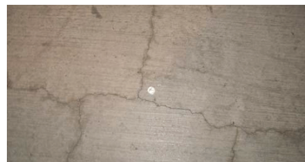
Fig. 8 – When the original structure was built, the slabs made with portland cement concrete exhibited drying-shrinkage cracking before the concrete was strong enough for post-tensioning.
