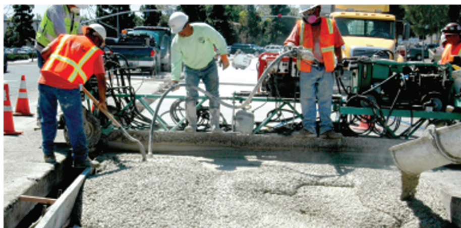
Fig 3 - Panel replacement work on Highway 1 in San Luis Obispo, Calif.
