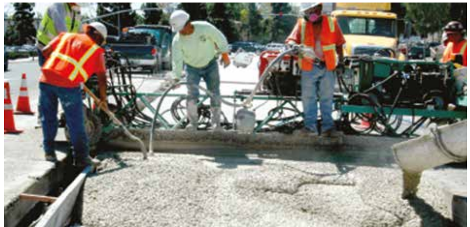
Fig 3 - Panel replacement work on Highway 1 in San Luis Obispo, Calif.
