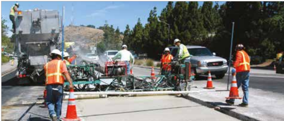
Fig 1 - Panel replacement work on Highway 1 in San Luis Obispo, Calif.
