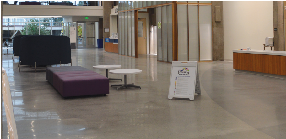
Fig 1 - Plans called for 22,000 square feet of flooring on two floors to be topped with Rapid Set® TRU® PC by CTS Cement.
