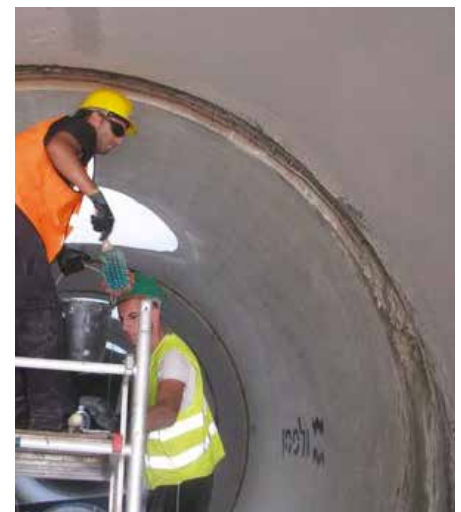
ISRAELI POWER PLANT: Cement All was used on connections between pipes.
