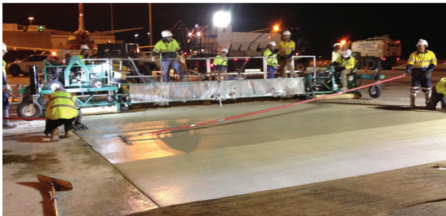
SYDNEY INTERNATIONAL AIRPORT: They only had six hours working time and replaced pavements needed to be strong enough by 5 a.m. to handle aircraft traffic loading.
