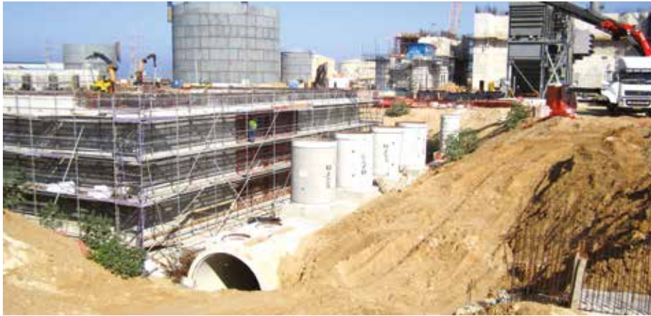
ISRAELI POWER PLANT: To avoid having any weak points in the piping for the Dorad Power Plant in Ashkelon, Israel, careful attention was paid to the connection between pipes. Instead of using portland cement grouting for this application, Rapid Set Cement All was used - a high performance blend of Rapid Set Cement and specialty sand.
