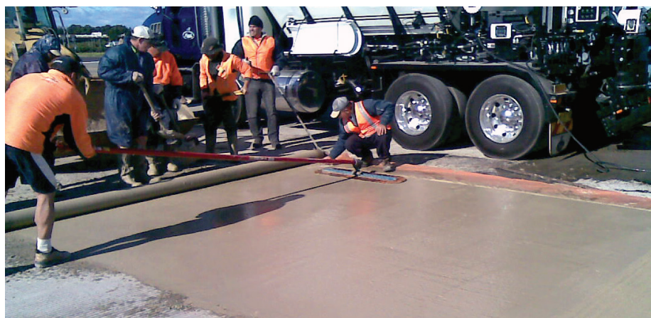
To minimize disruption to air traffic and scheduling at this heavily traveled Sydney International Airport, the crew worked only at night to repair damaged slabs. They only had six hours working time and replaced pavements needed to be strong enough by 5 a.m. to handle aircraft traffic loading.
