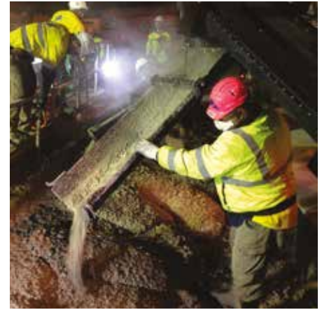
SYDNEY INTERNATIONAL AIRPORT: all 12 of the damaged slabs were replaced within 10 working days.
