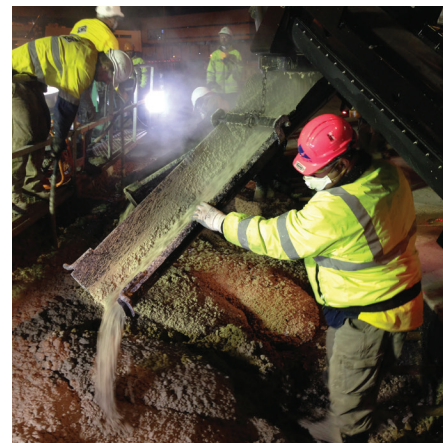
SYDNEY INTERNATIONAL AIRPORT: all 12 of the damaged slabs were replaced within 10 working days.
