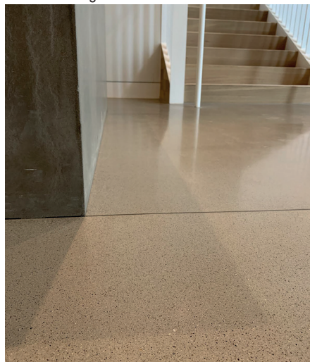
This office lobby in Austin, Texas, is finished with Rapid Set® TRU® SP. The high-performance, self-leveling architectural topping has undergone extensive testing of its comprehensive, tensile and flexural strengths to provide a more comprehensive analysis of its overall performance when it comes to cracking.
