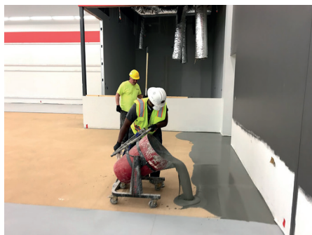
Maintain a wet edge when placing an overlay.
