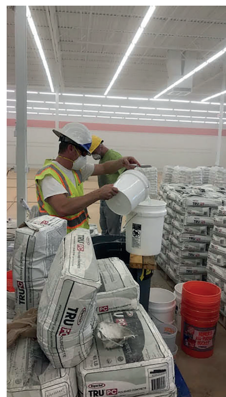
Use proper mix proportions to keep aggregate suspended and near the top of the surface,
