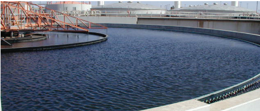
In El Paso, Texas, Type K cement was used in the construction of two treatment plants, which are still virtually crack-free almost 20 years after they were built. This is no small feat in a city where high heat, low humidity, and sizeable temperature swings create less-than-ideal conditions for concrete structures.
