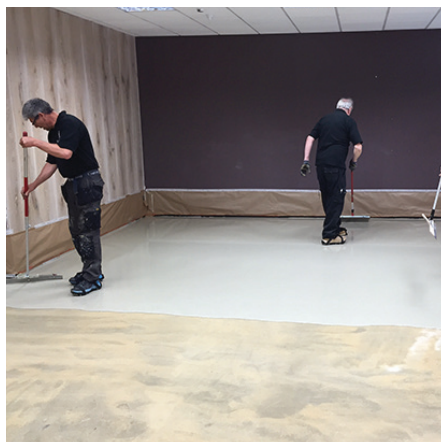
Top: Contractors installing a CSA cement-based self-leveling topping. The one-component system was poured at a depth of 12 mm and cured for 24 hours. Bottom: The floor was finished with two coats of acrylic polish and burnished with a white pad to achieve a high gloss. Photos courtesy of STM LTD.
