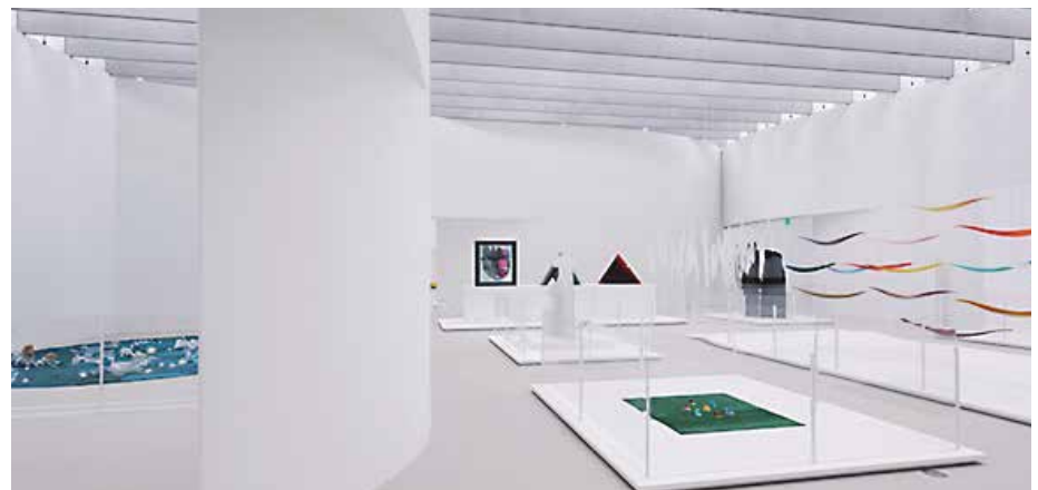
The architect wanted an extremely light gray concrete floor for subtle contrast to the bright-white plaster walls. A CSA cement-based topping was combined with integral coloring, and polished to a low sheen.
