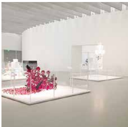
The one-component CSA cement-based topping system cures to a light off-white color, and may be stained, dyed or integrally colored. Adding custom pigment achieved a very light gray that was perfect for the light-filled space.
