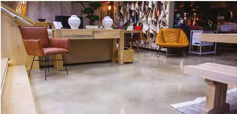
This beautiful concrete floor was finished with a two-tone, cloudy look and polished to a high shine. Contractors completed the work in just three days, using CSA cement-based products. Photo courtesy of Specialised Tools & Machinery (STM) LTD.
