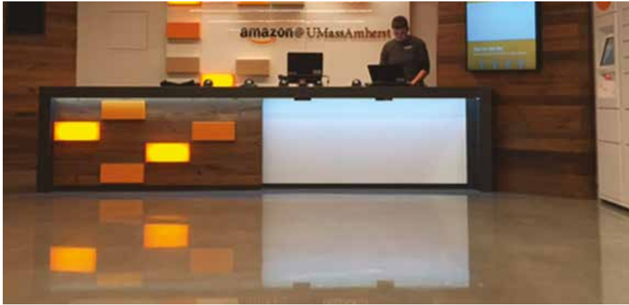
The distribution center's contemporary, polished concrete floor is subject to foot traffic in the ordering area, as well as pallet jacking in the supply room.
