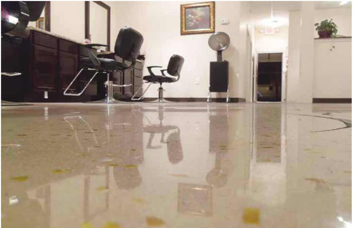
Fig 3 - The floor was seeded with mirrors, as well as amber, red and yellow aggregates.
