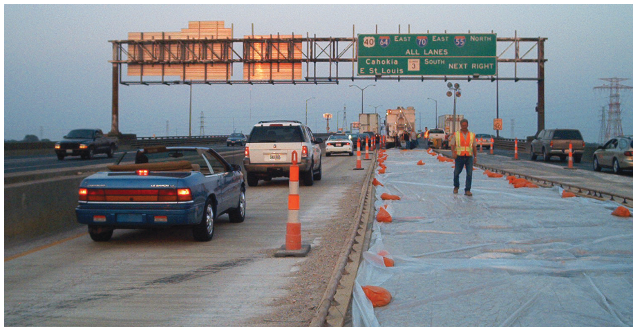
Highway J Bridge
