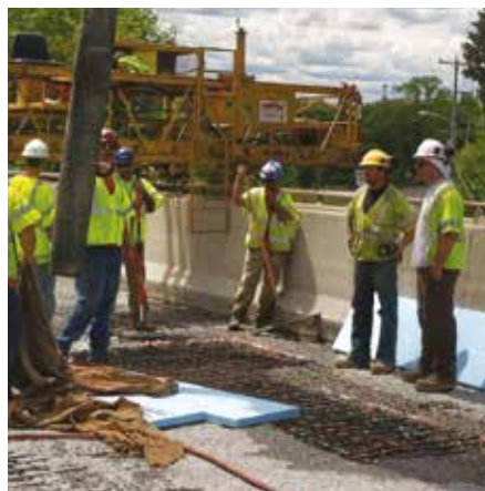
Route 95 Bridge Rehabilitation
