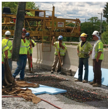
Route 95 Bridge Rehabilitation
