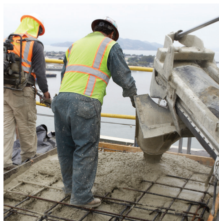
San Francisco-Oakland Bay Bridge
