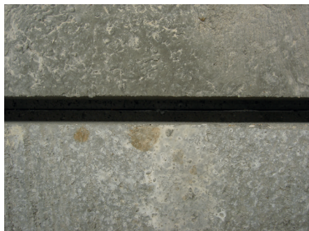
Pictured is a top view of a keyway joint.
