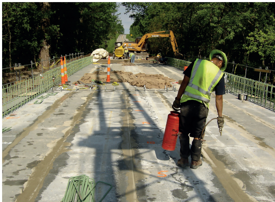
The contractor sprays a curing compound on the keyway joints.
