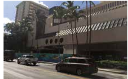
As part of this renaissance, the Waikiki Trade Center—an underused 22-story office and retail building—is being transformed into an upscale, 230-room by Swinerton Builders Hawaii. This hotel will include street-level retail space, and specialty fashion retailer Nordstrom Rack will be one of its first tenants.
