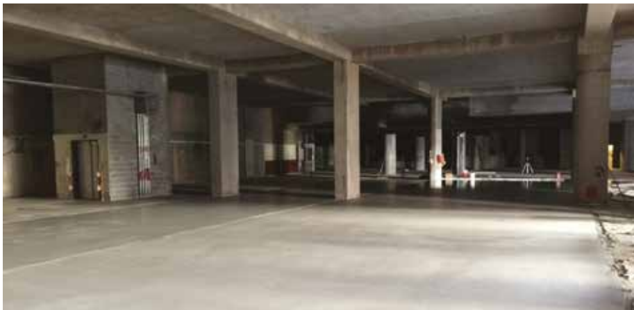
Nordstrom specified Rapid Set® Products for the overlay, which included LevelFlor® self-leveling underlayment, TXP™ Epoxy Primer and TRU® Self-Leveling topping. CTS RAPID SET
