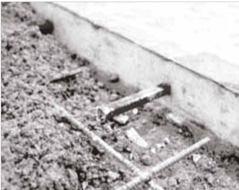
Fig. 6 – Square dowels with special clips (red) having cushioning side pads to allow differential horizontal movements but transfer vertical loads. Note: optimized concrete mixture that appears harsh and “stony” but is actually extremely workable and finishable.
