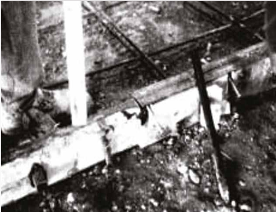
Fig. 4 – Prefabricated system consisting of steel angle armored floor construction joint, edge forms with and without armor angles, reusable dowel holders/aligners (red), etc. As adjacent slab panels shrink away from joint, elastomeric adhesive between two angles allows them to separate.
