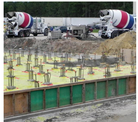
Fig. 2 – This slab was placed on 535 augercast piles and was tied to the piles with reinforcement extending out of the piles and hooked into the slab.
