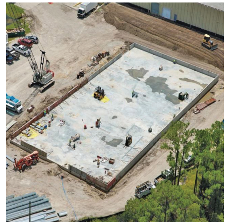
Fig. 4 – The foundation consists of a mat slab that is 102x206 ft. and 32 in. thick. The engineer's main concern was that there could be no control or construction joints in the slab. To achieve this, the engineer chose CTS Cement's KSC Komponent.
