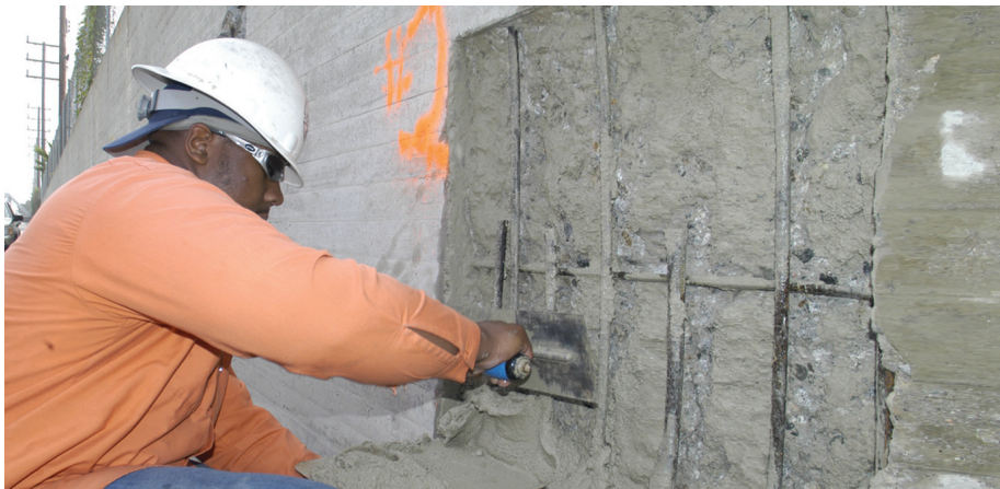
Fig 1 - Exterior wall repair.
