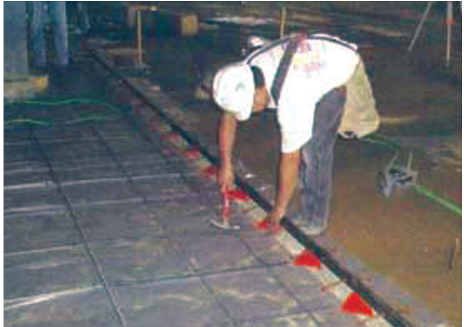
Fig. 3 – The plate dowel pocket former is nailed to the form prior to casting the first slab.
