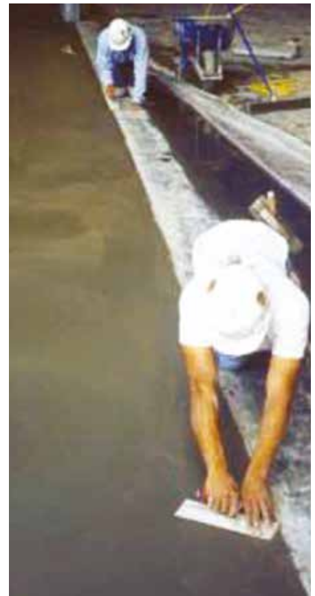
Fig. 2 – Hand troweling of the joints ensures that the joints are flat.
