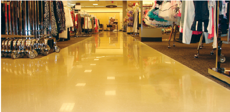
Fig 1 - The Nordstrom Rack clothing store in Aventura, Fla., contains 7,000 square feet of polished overlay, including this aisle. The project is the work of Creative Concrete Services, Lakeland, Fla.
