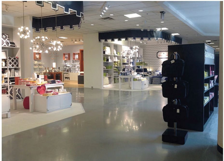
Fig 3 - Each night, the merchandise is covered before work can begin on the "streets" in this JCPenney store at West Towne Mall in Madison, Wis. This particular job features CTS Cement's Rapid Set TRU overlay.
