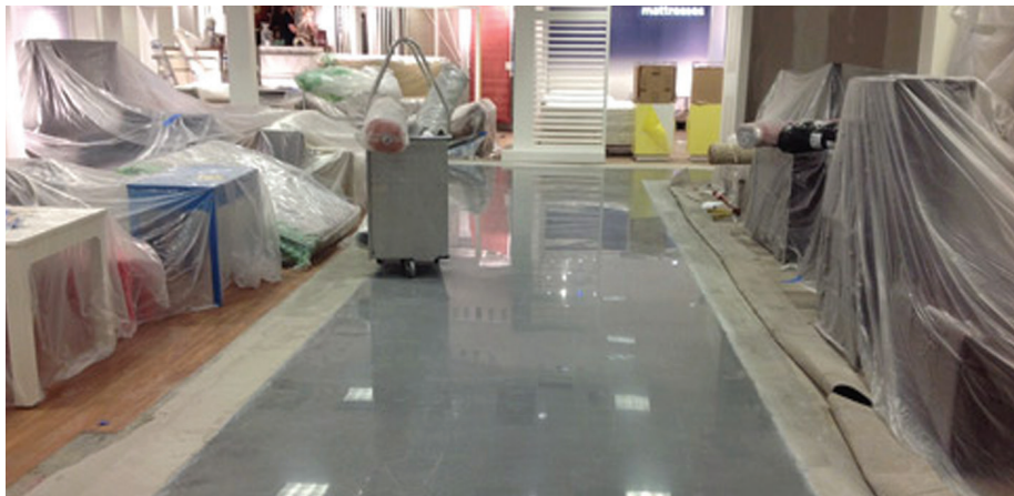
Fig 1 - Each night, the merchandise is covered before work can begin on the "streets" in this JCPenney store at West Towne Mall in Madison, Wis. This particular job features CTS Cement's Rapid Set TRU overlay.
