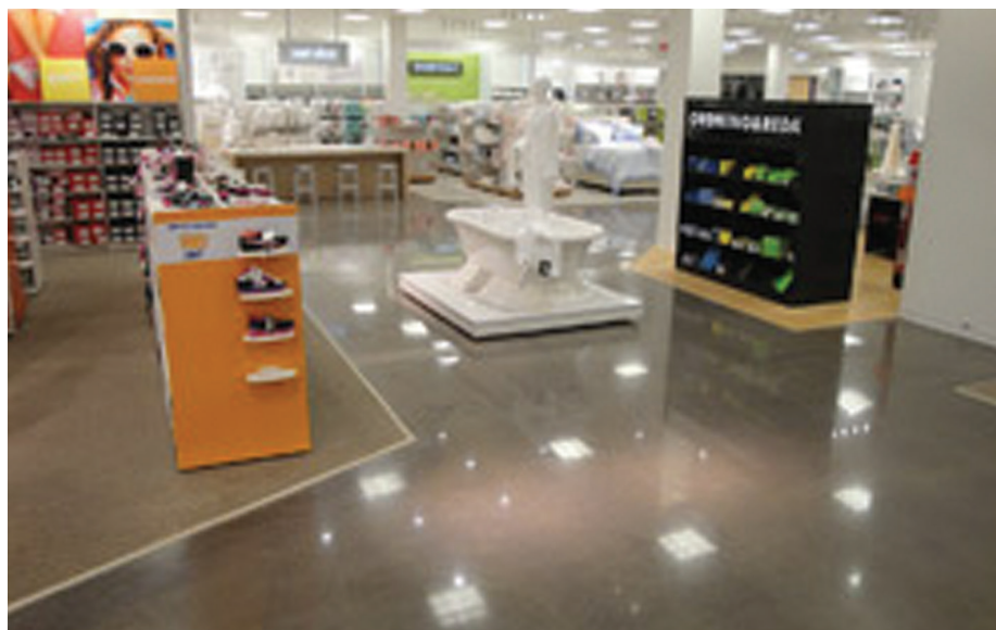
Fig 6 - In this stand-alone store in Canton, Mich., the contractor polished the existing underlayment, but all the joints had to be rebuilt with Rapid Set TRU. It was a massive repair project.
