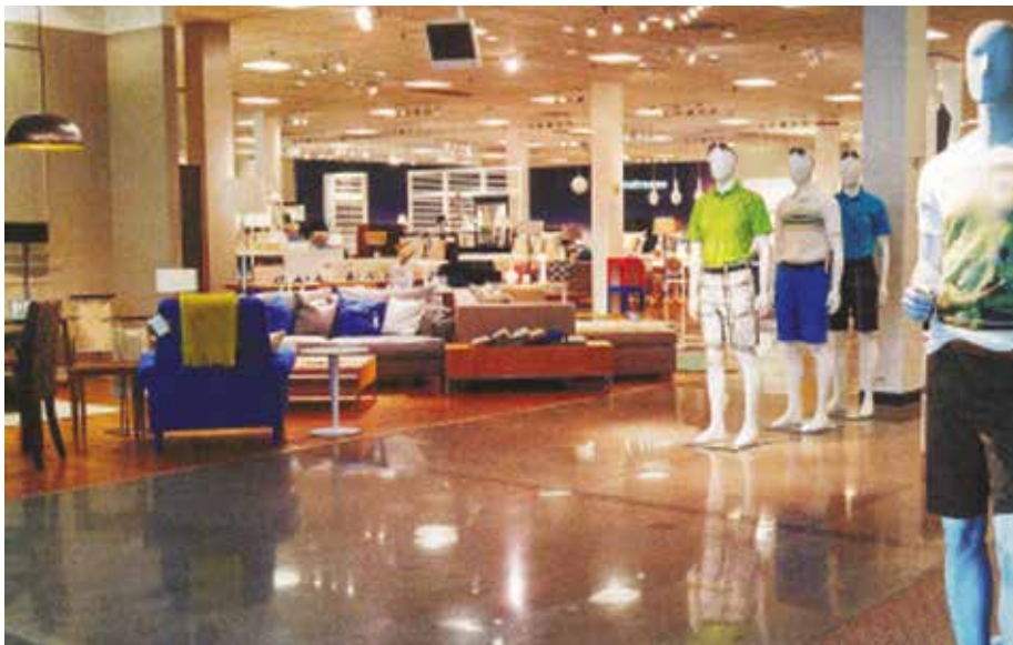
Fig 5 - A large area of the Merrillville, Ind., store was remodeled in the recent waves. With the lighting in place, the newly polished streets really pop. Rite-Way Concrete Seal Systems, Wolcott, Ind., served as the contractor.
