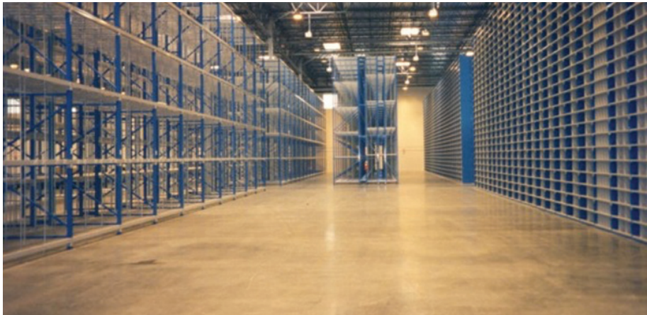
Fig. 1 – The Toyota Parts Center, Ontario, Calif. is a super flat floor with joint spacing up to 120 ft.
