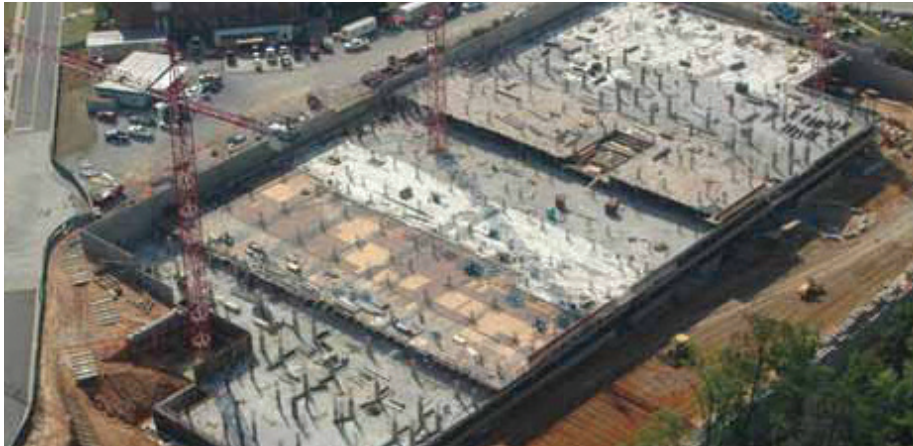
Fig. 1: Aerial view of Ridgecrest South under construction on May 20, 2008. The slab-on-ground is complete, and more than half of Level 1 and one-third of Level 2 have been cast
