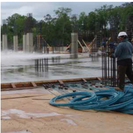
Fig. 4: For the elevated slabs in the garage levels, fogging was started immediately after concrete placement
