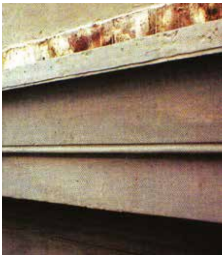
Close-up of repaired area on walls: after
