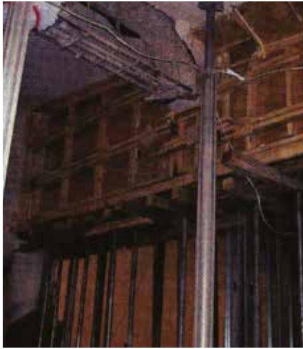
View of the full-depth beam repair
