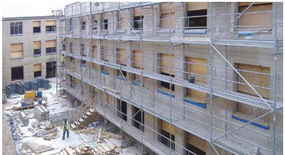
View of interior lightwell work area
