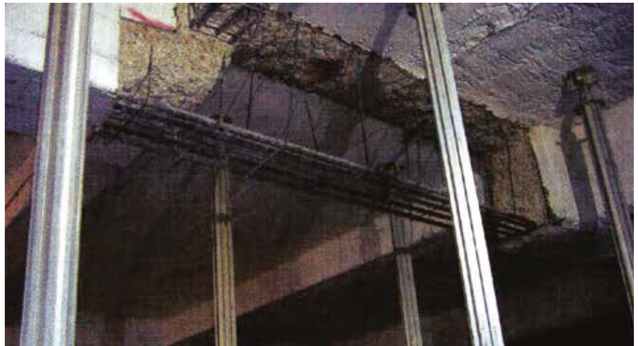
Interior beam repair work – notice the extensive shoring
