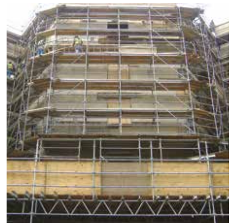
Repair crews working on Pentagon walls
