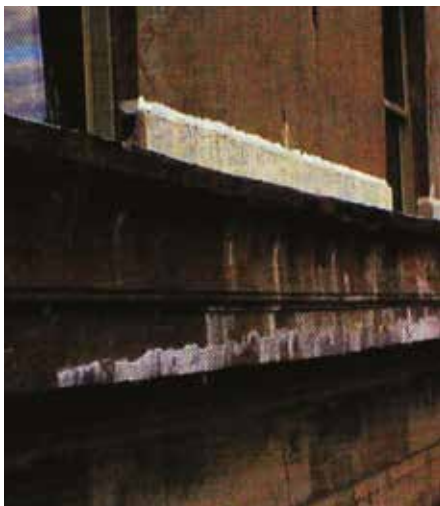
Close-up of repaired area on walls: before
