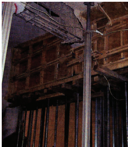
View of the full-depth beam repair
