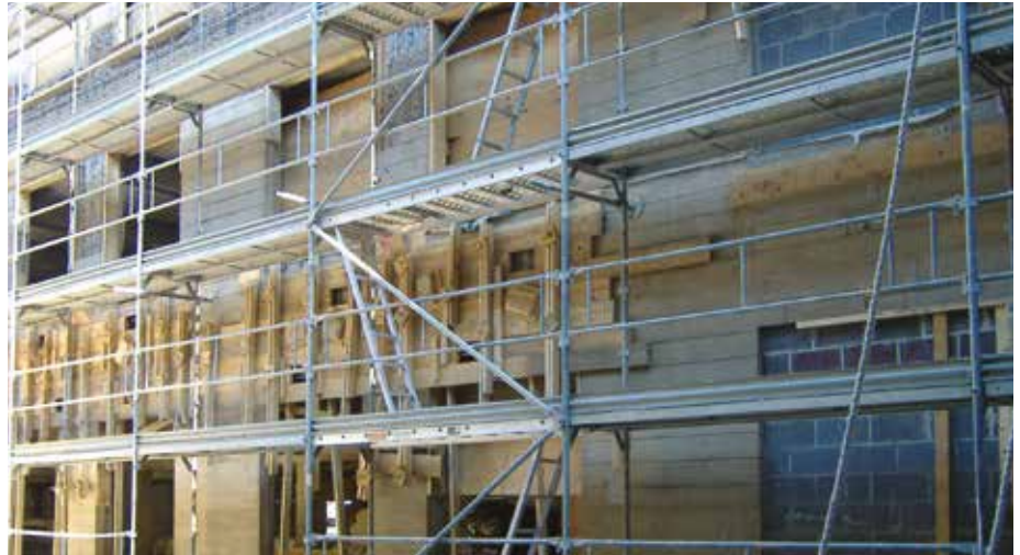
Work area showing extensive scaffolding
