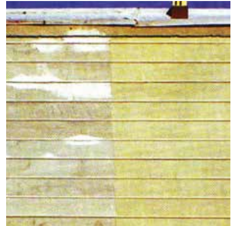
Before and after coating application
