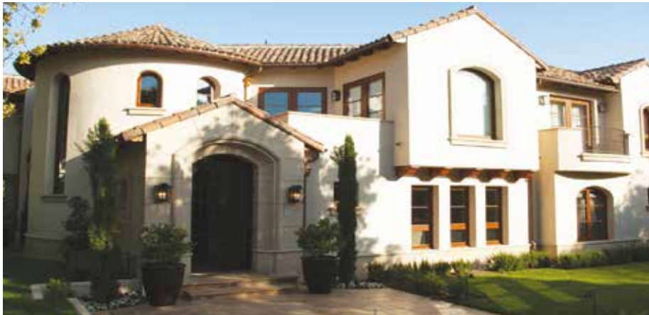
Fig 1 - Design professionals can obtain the benefits of a genuine plaster finish by using rapid-setting plaster based on calcium aluminosulfate cement.
