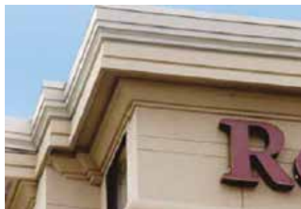
Fig 5 - In extreme weather environments, rapid-setting plaster can provide the beauty and durability of a traditional plaster finish while minimizing the risks and costs associated with portland cement plastering.
