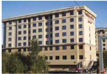
Fig 3 - Nine months after plastering was completed, the general contractor on the Marriott Hotel project reported an excellent finish with no cracking. The use of calcium aluminosulfate (CAS) cement was a success. Photo courtesy Ferguson Construction
