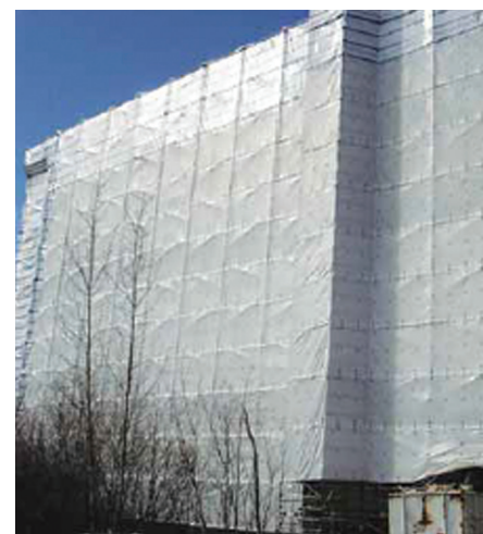
Fig 2 - This eight-story Marriott Hotel project was plastered during the winter in Bellevue, Washington. Due to near-freezing conditions and the heavy rain common to the region, it was tented to protect both plaster and plasterers. Rapid-setting plaster was used, so overnight heating was not necessary.
