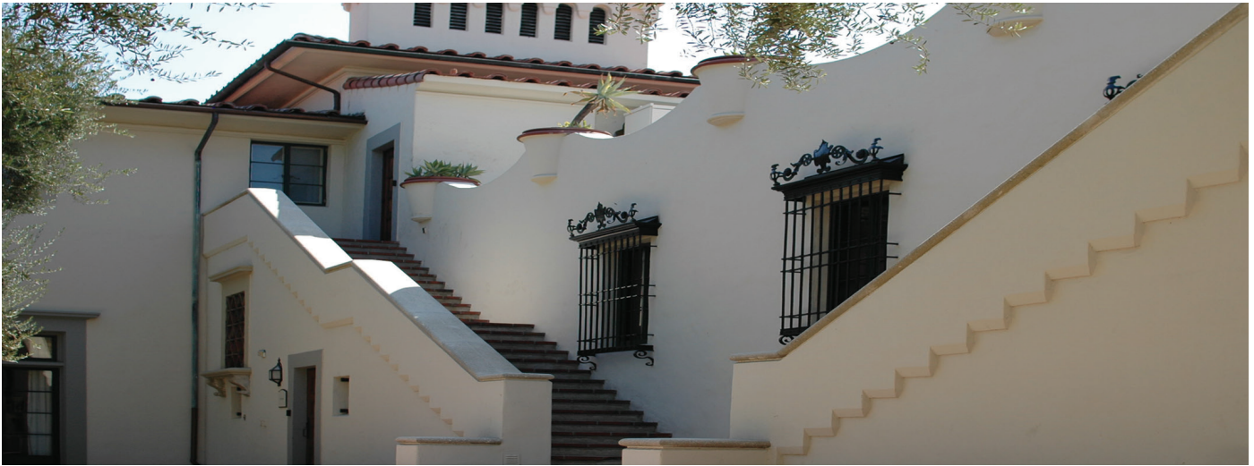
Fig 2- High-performance rapid-setting cement helped replace a number of badly weathered concrete stairways.
