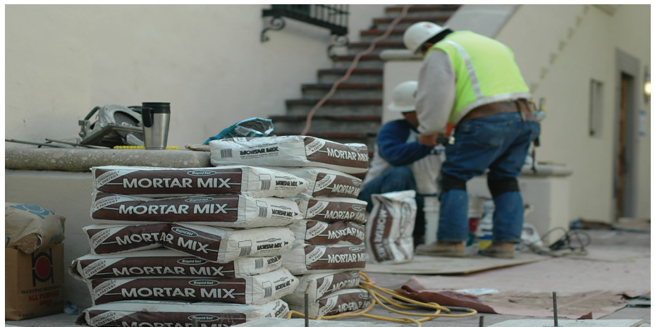
Fig 4- Crews used Rapid Set® Mortar Mix to match the original look with addition of dry powder pigments and specifically composed aggregate mixes.
