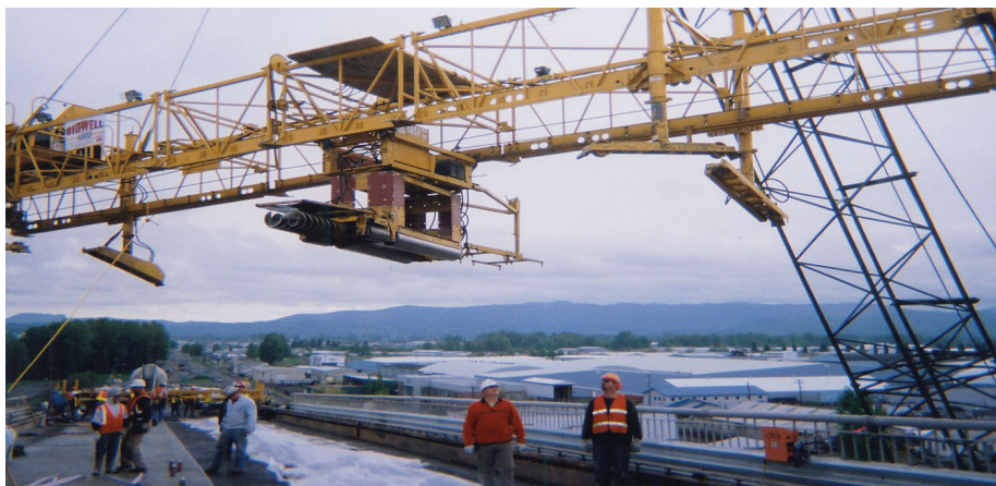
Fig. 1 – While some sections of the historic Lewis & Clark bridge had to be completely replaced, much of the deck could be refurbished by applying a new concrete overlay. The repair will extend the life of the span another 25 years.
