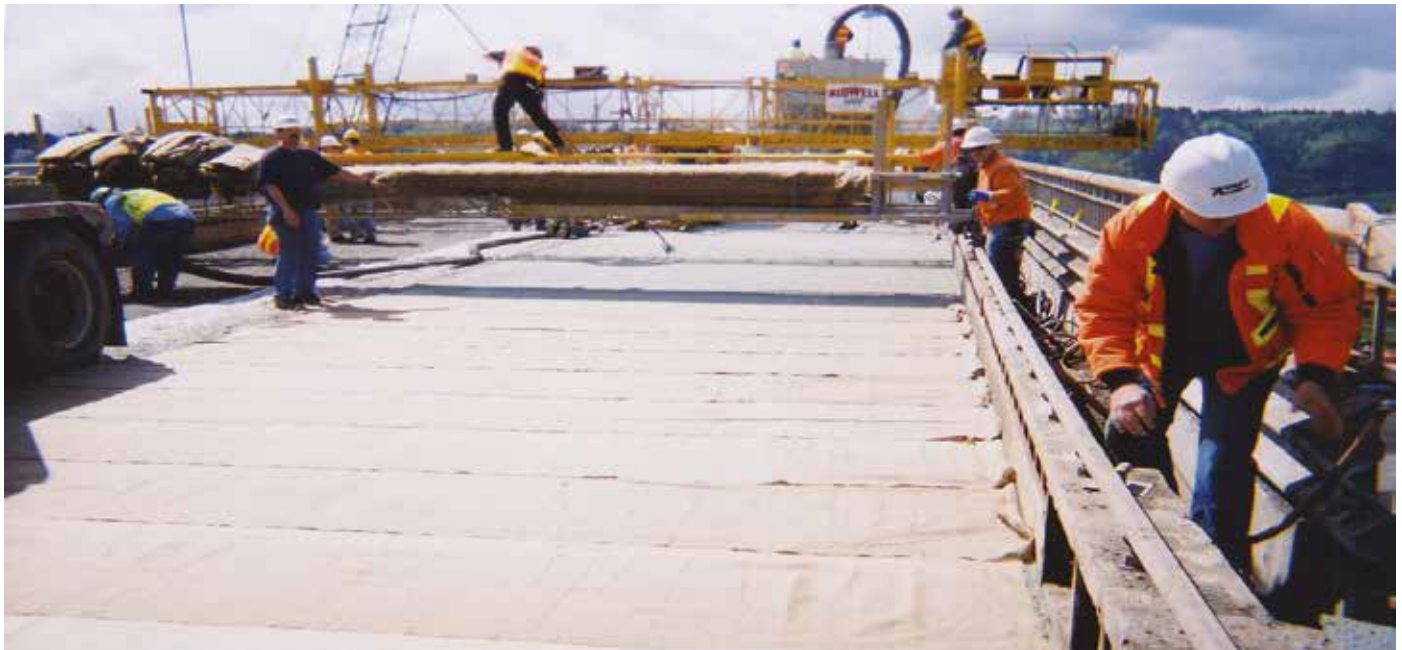
Fig. 2 – The repairs were finished a full 10 days ahead of schedule.
