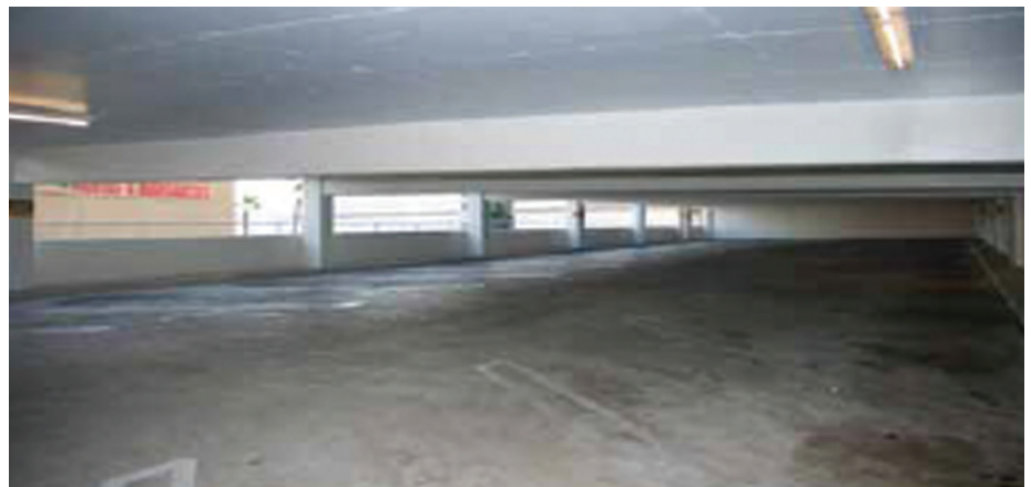
Fig. 4 – Beam and Slab Framing (4 th Level)
