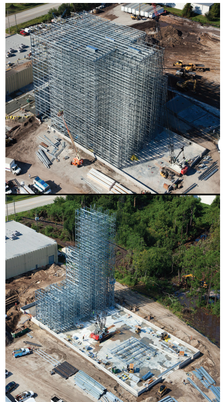
Fig. 2 – The foundation consists of a mat slab that is 102-feet by 206-feet and 32 inches thick.
