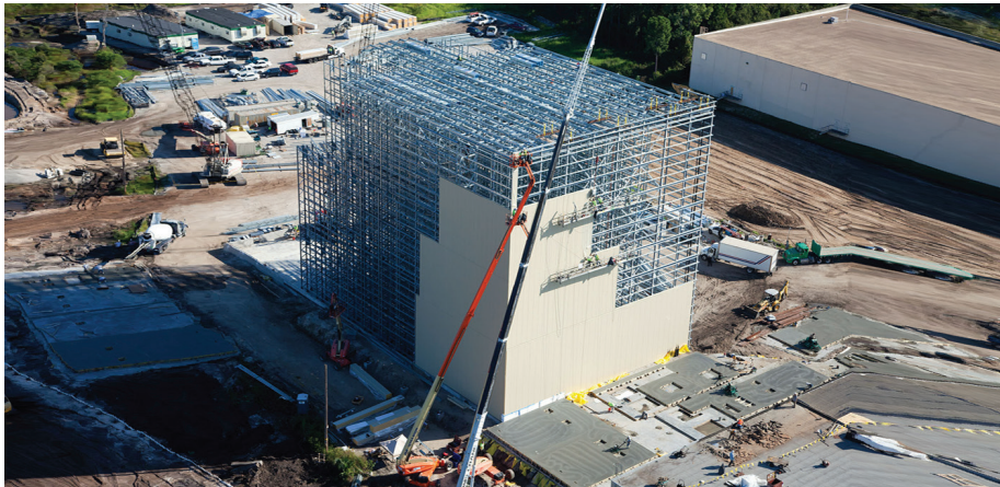
Fig. 1 – The low bay has a typical clearance height of 30 feet but the high bay is 115 feet tall, which is a remarkable 10 stories.
