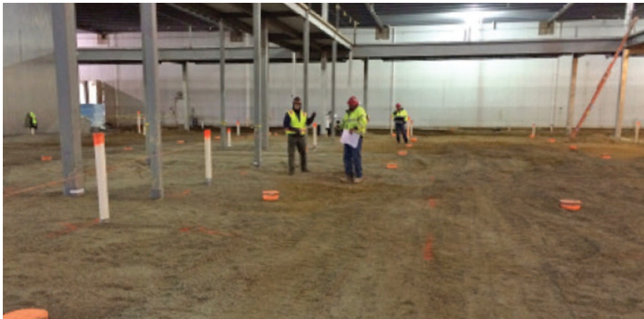
Fig. 1 – One of the major concerns on the project was the extensive plumbing running throughout the floors with a potential for reflective cracking along the pipe placements. Photo Credit: CRT Concrete Consulting.
