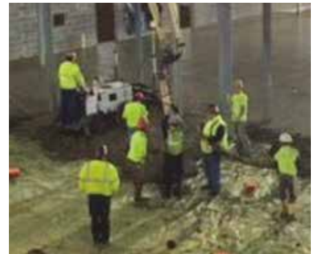
Fig. 3 –After much consideration the contractor chose to utilize a Somero S-840 Laser Screed® machine equipped with the Somero 3-D Profiler System®. The S-840 offered the proper screed head width and was also equipped with a 3D blade to fine-grade the sub-base to accurately control concrete thickness and yield. Photo Credit: CRT Concrete Consulting.
