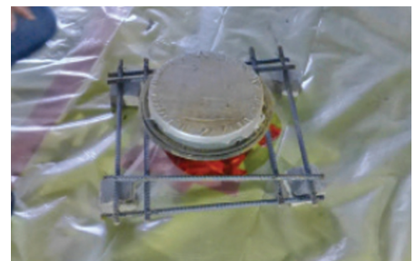
Fig. 4 –The only steel required was two #4 bars at the perimeter of each pour and around columns or other penetrations. Photo credit: CRT Concrete Consulting
