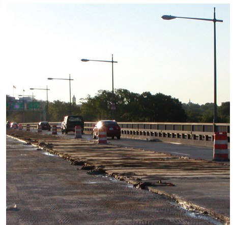
The Theodore Roosevelt Bridge in Washington, D.C. is being repaired with Rapid Set® latex modified concrete. Photos: CTS Cement Manufacturing Corp.
