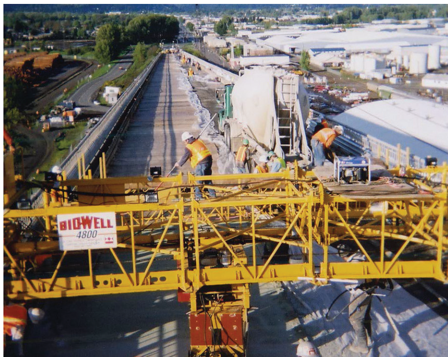
Rapid Set® cement is being used for the overlay of the 79-year-old Lewis and Clark Bridge over the Columbia River between Washington and Oregon.
