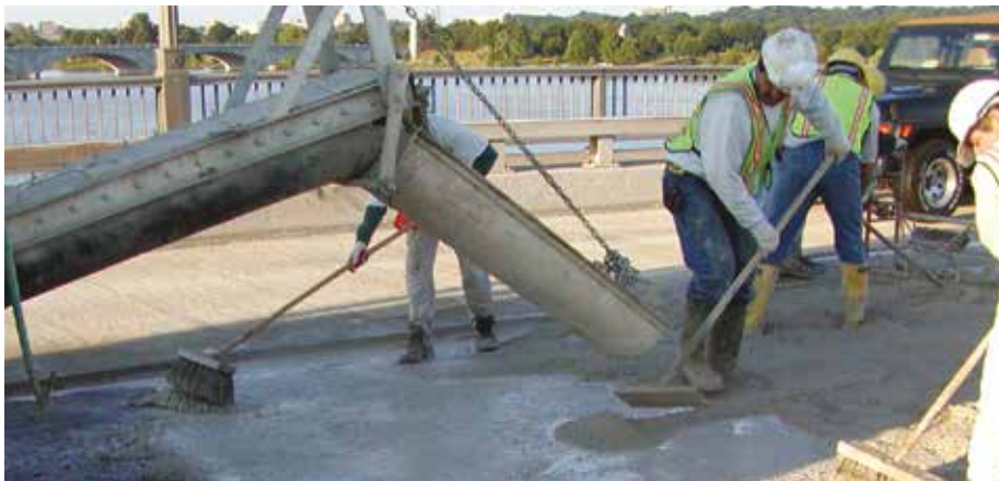
The Theodore Roosevelt Bridge in Washington, D.C. is being repaired with Rapid Set® latex modified concrete. Photos: CTS Cement Manufacturing Corp.
