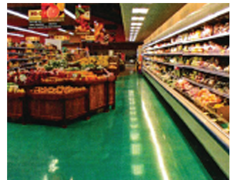
Fig 2 - TRU® Self-Leveling was mixed with Ameripolish OS Dye to produce the green color for the produce section.
