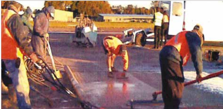
Fig. 1 – Rapid-setting concrete offers technological advances for spall, crack and crater repairs on military airfields.
