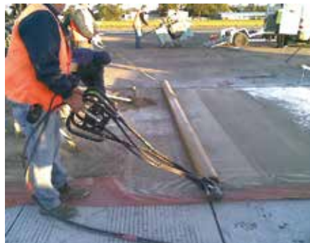
Fig. 5 – Placing and finishing of a slab.
