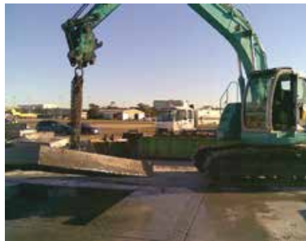
Fig. 3 – New, faster method of slab removal.
