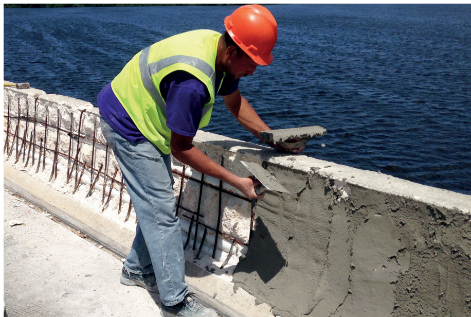
Teodoro Moscoso Bridge, San Juan, Puerto Rico, repairs of side barriers and drain basins, partial-depth concrete pavement repairs using Rapid Set® Cement All®, Mortar Mix, V/O Repair Mix, WunderFixx®, CR Concrete Resurfacer, DOT Repair Mix, and Corrosion Inhibitor.
