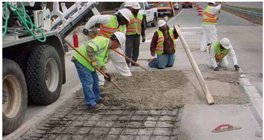
Fig. 6 – Virginia DOT repairs.
