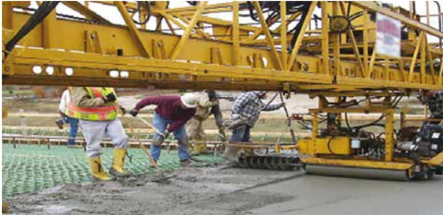
Fig. 1 – Crews use rapid-setting cement for the deck overlay of the M6 Beltway project in Grand Rapids, Mich.
