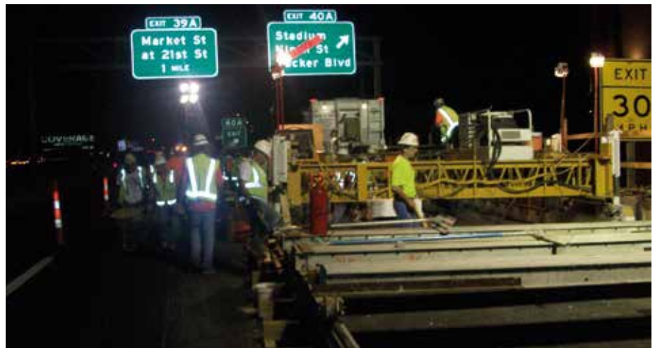
Fig. 5 – Missouri DOT emergency repairs to the Busch Stadium on-ramp.
