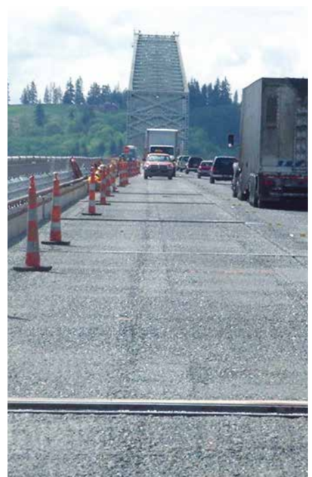
Fig. 2 – Completed Lewis and Clark Bridge open for traffic.
