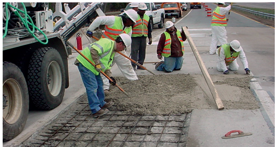
Fig. 6 – Virginia DOT repairs.
