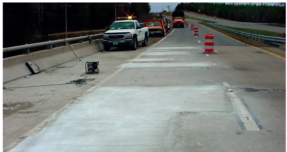
Fig. 7 – Virginia DOT highway repairs, Mecklenburg County
