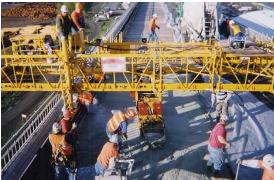
Fig. 4 – Crews working on the Lewis and Clark Bridge
