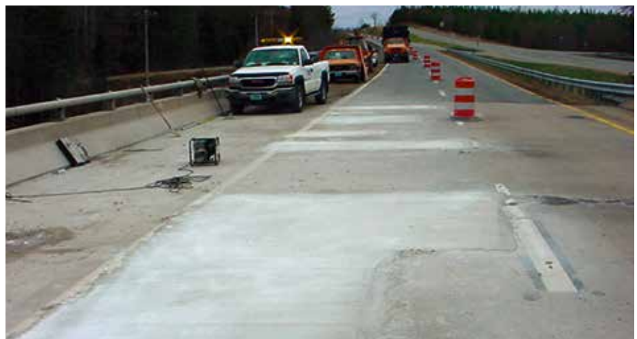
Fig. 7 – Virginia DOT highway repairs, Mecklenburg County
