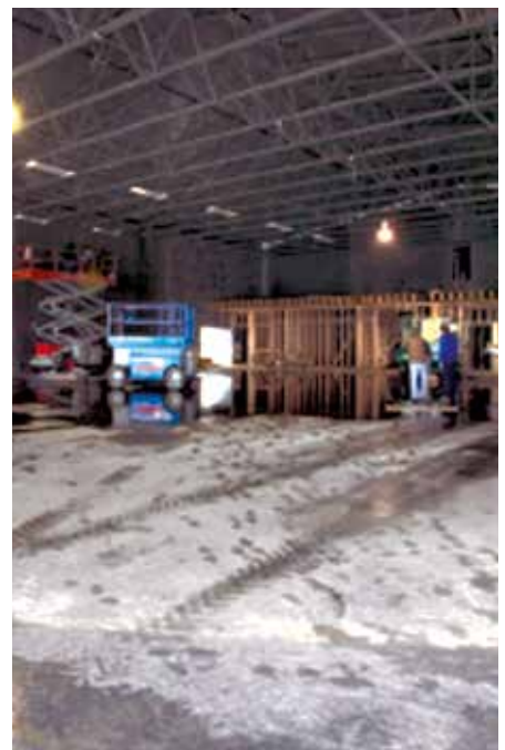
Fig. 2 – Health and safety can be concerns in certain traditional concrete floor applications. For example, heavy forklifts used in warehouses can cause individual slabs to move up and down over time, creating a bump. Shrinkage-compensating concrete does not require the use of control joints.
