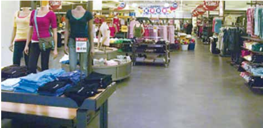
Fig. 1 – Type K cement was used to produce a crack-free concrete floor at an Old Navy store in Portland, Oregon. The space's previous floor had failed due to cracking. Based on this experience and unsuccessful refinishing, the owner requested the use of joints in the replacement floor.
