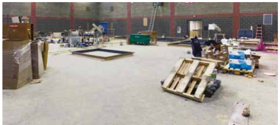
Fig. 4 – Shrinkage-compensating concrete is made with a small percentage of Type K expansive cement, which causes the concrete to expand before it dries, relieving the tensile stresses caused by drying shrinkage. As such, it can prevent cracks and achieve a jointless floor.
