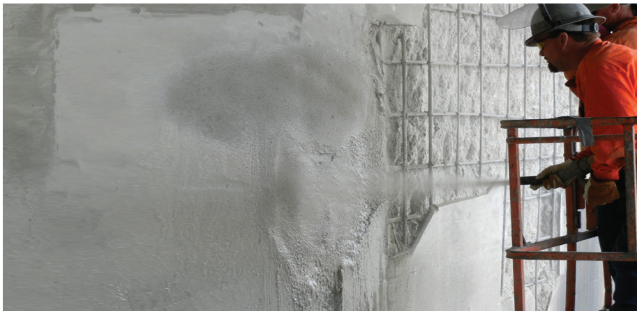
Fig 1 - Calcium Sulfoaluminate (CSA) cement exhibits properties uniquely suited to the harsh environment of underground construction.
