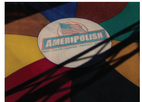
Fig 5 - This detail from the AmenPohsh booth at World of Concrete 2013 was done using CTS Cement's Rapid Set TRU Self Leveling and shows eight different integral colors. The central circle is TRU without integral color. The logo, dyed with a two-layer laser-cut stencil, is about 18 inches across.
