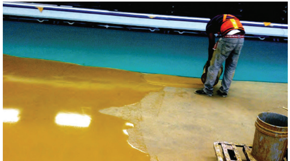
Fig 3 - After one color is poured and has cured, the foam strips are removed and the second color can be cleanly butted up against the first.
