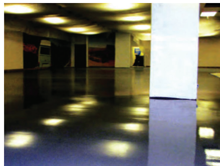
Fig 4 - The self-leveling overlay forms a thin, but extremely durable layer. It is often harder than the original concrete, which provides an ideal surface for polishing.
