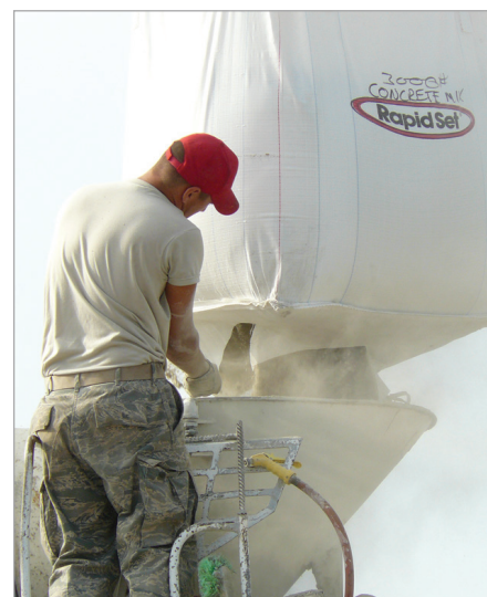
Fig. 2 – Rapid-setting concrete comes in both bag and bulk.
