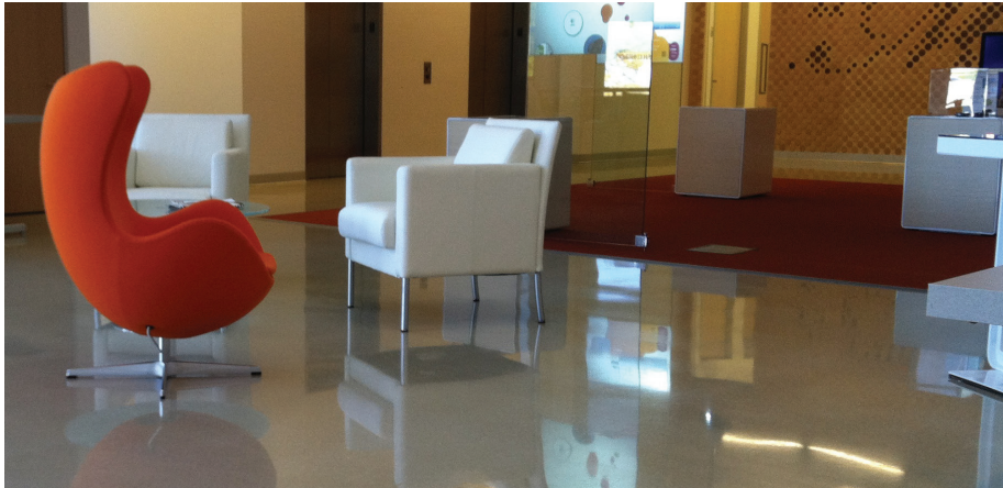
Concrete Visions installed a 5,200 ft 2 polished overlay at a corporate training center in Plano, Texas. Mirrored-glass aggregate captures light and makes the floor twinkle.
