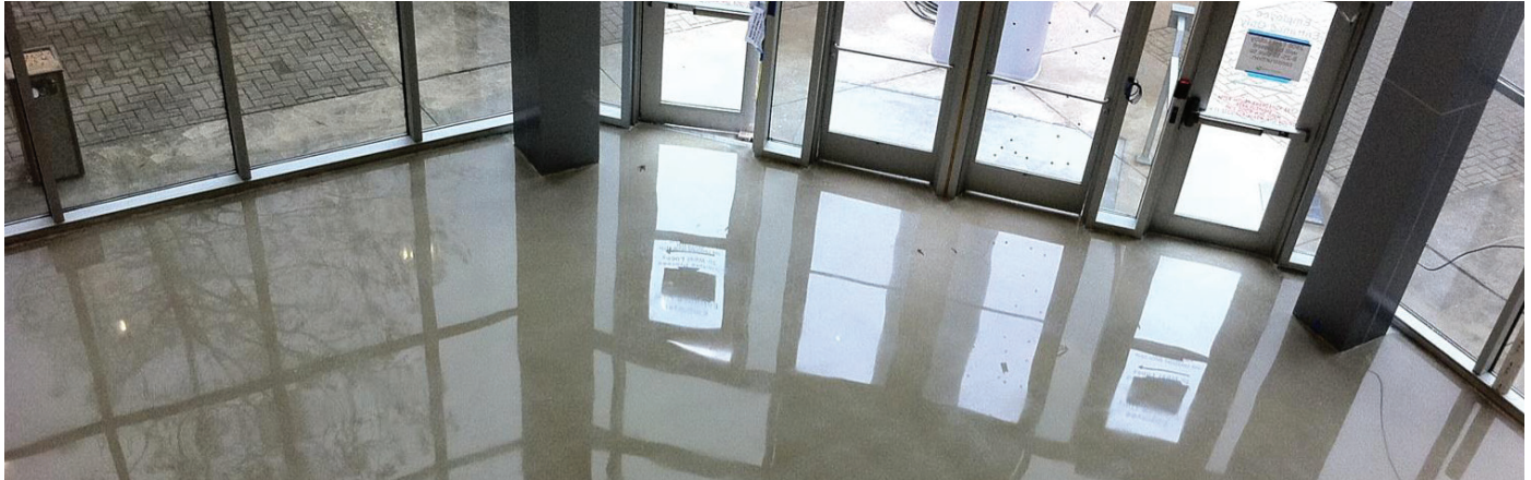
In order to prevent unwanted scratches, the Concrete Visions crew cleaned the floor between each abrasives step to remove any particles left behind from the polishing process.
