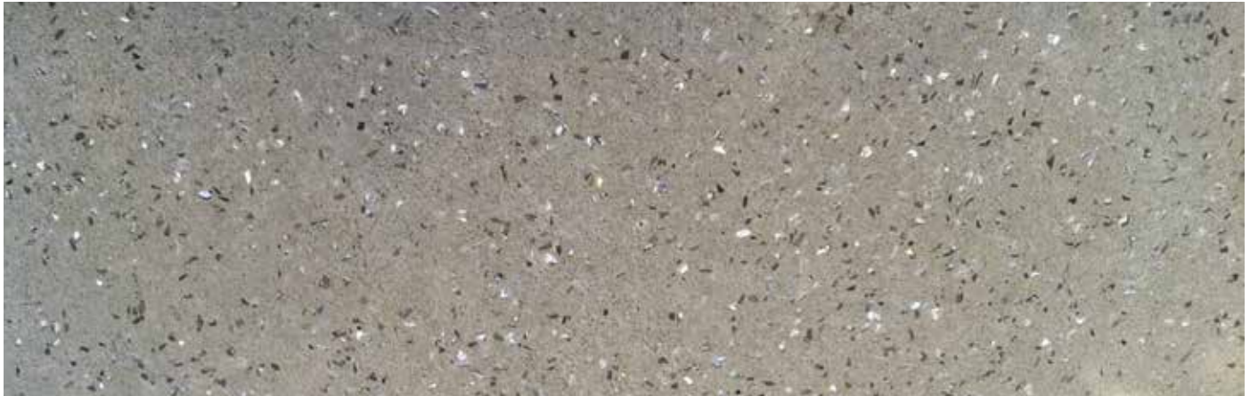
Roy Bowman, president of Concrete Visions, broadcasts mirrored-glass aggregate chips 1/8-inch and smaller on top of a concrete overlay.
