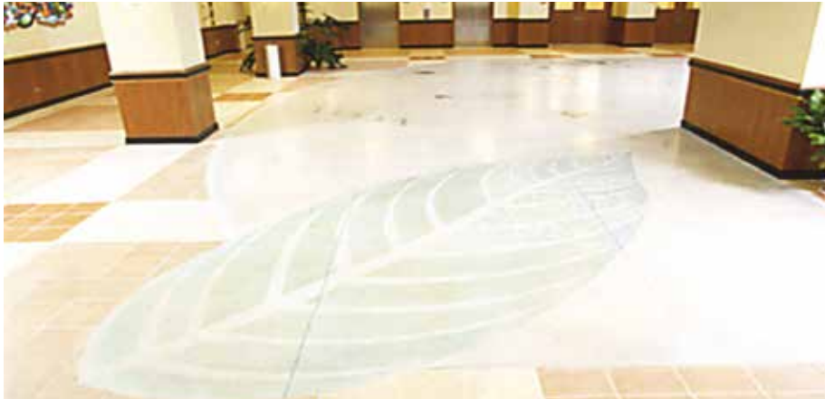
Among the polishable overlays on the market today are several featuring cement-based systems, such as the Mosaic topping manufactured by LifeTime Floors. The topping is designed to be applied wet on between 1/2 inch thick on freshly poured concrete slabs. After it's cured, it should be ground down and taken up to a full polish. Seen here is a Mosaic floor at the University of Texas, San Antonio.
