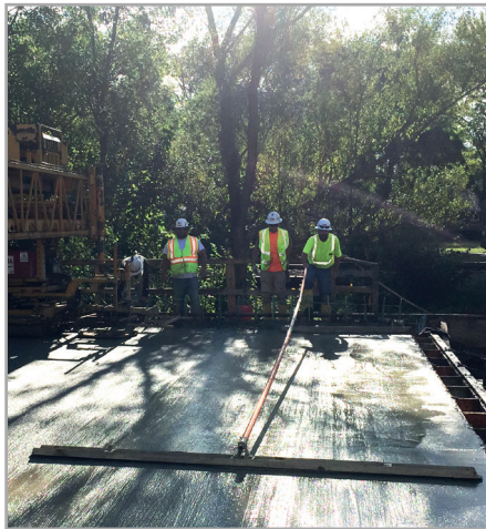
Figure 3 – Workers using a bull float to apply a smooth finish to the Type K cement concrete pavement.
