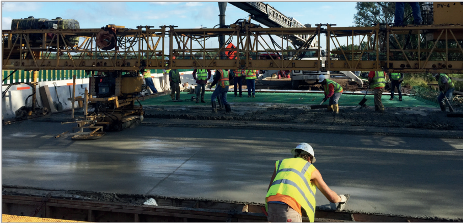
Figure 1 – Stark Excavating places and finishes a Type K cement concrete bridge deck in Peoria, Illinois, over Boyd's Hollow Creek on Route 29. Concrete was supplied by VCNA Prairie.
