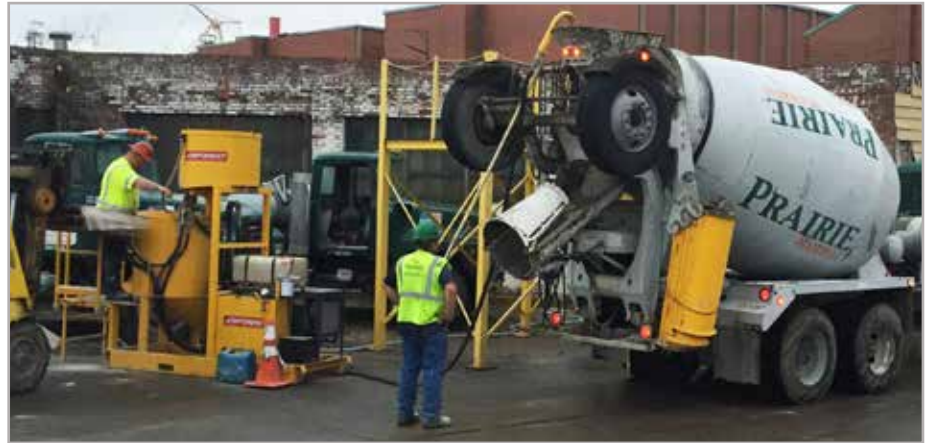
Figure 2 – CTS Cement Manufacturing's Komponent expansive cement additive is added using a ChemGrout slurry machine
