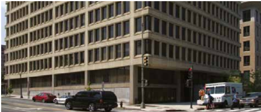
Fig. 1—500 First Street, NW is an eight-story building with two basement levels. Like many sites in the Washington, DC, area, there were significant groundwater issues to contend with in constructing the foundation. Erected in 1967, it was the first building in the city constructed with post-tensioning. (Photo by Steven H. Miller, courtesy of CTS Cement Manufacturing).
