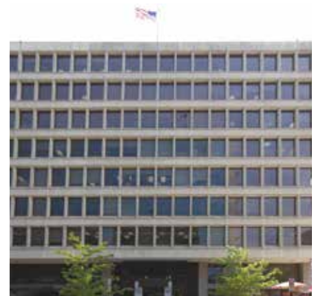
Fig. 5—Forty years later, the building is stable and in excellent condition. The thin deck-slabs made possible by posttensioning allowed the designers to get an extra story into the structure and still stay under the city's absolute height limit. The building is currently occupied by offices of the Federal Bureau of Prisons. (Photo by Steven H. Miller, courtesy of CTS Cement Manufacturing.)
